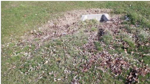
Excessive Sediment Buildup
