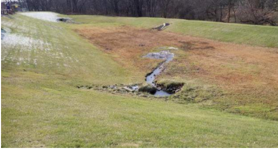
Detention Basin Erosion
