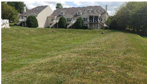
A: Dry detention basin
